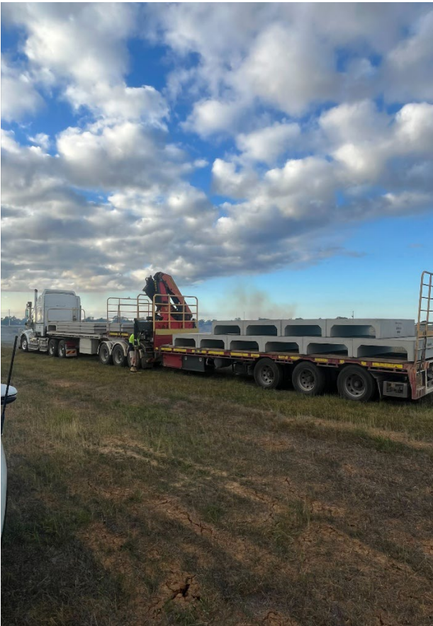
Delivery of box culverts to the Aerodrome heavy vehicle access site
