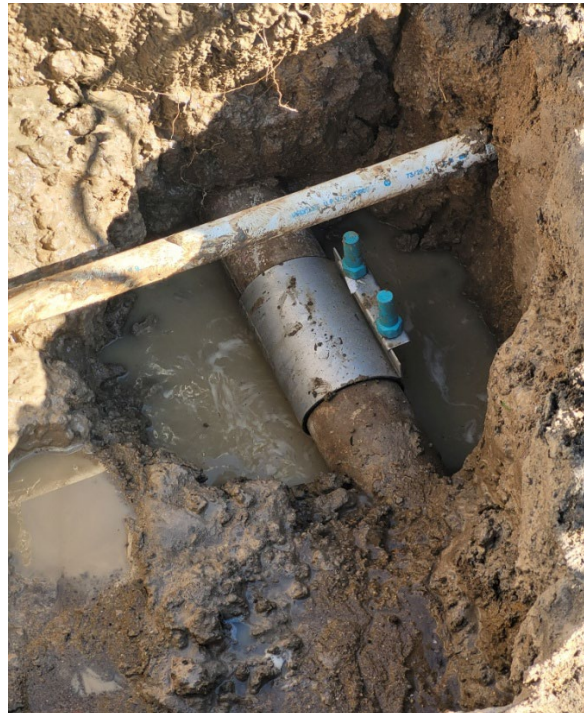
100mm Raw water main repair
