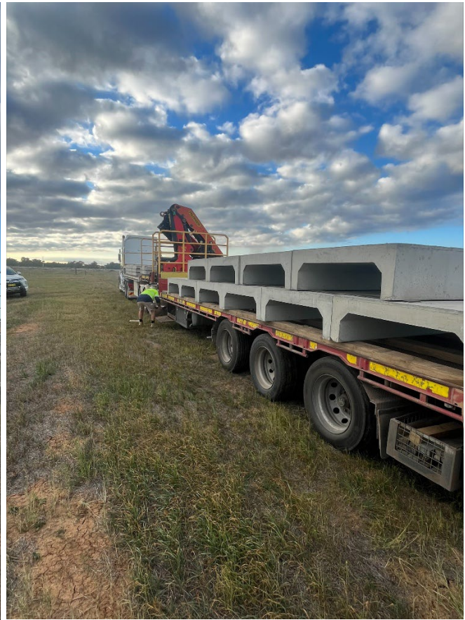
Delivery of box culverts to the Aerodrome heavy vehicle access site
