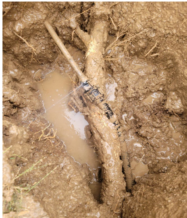
Filtered water service repair in Macauley Street
