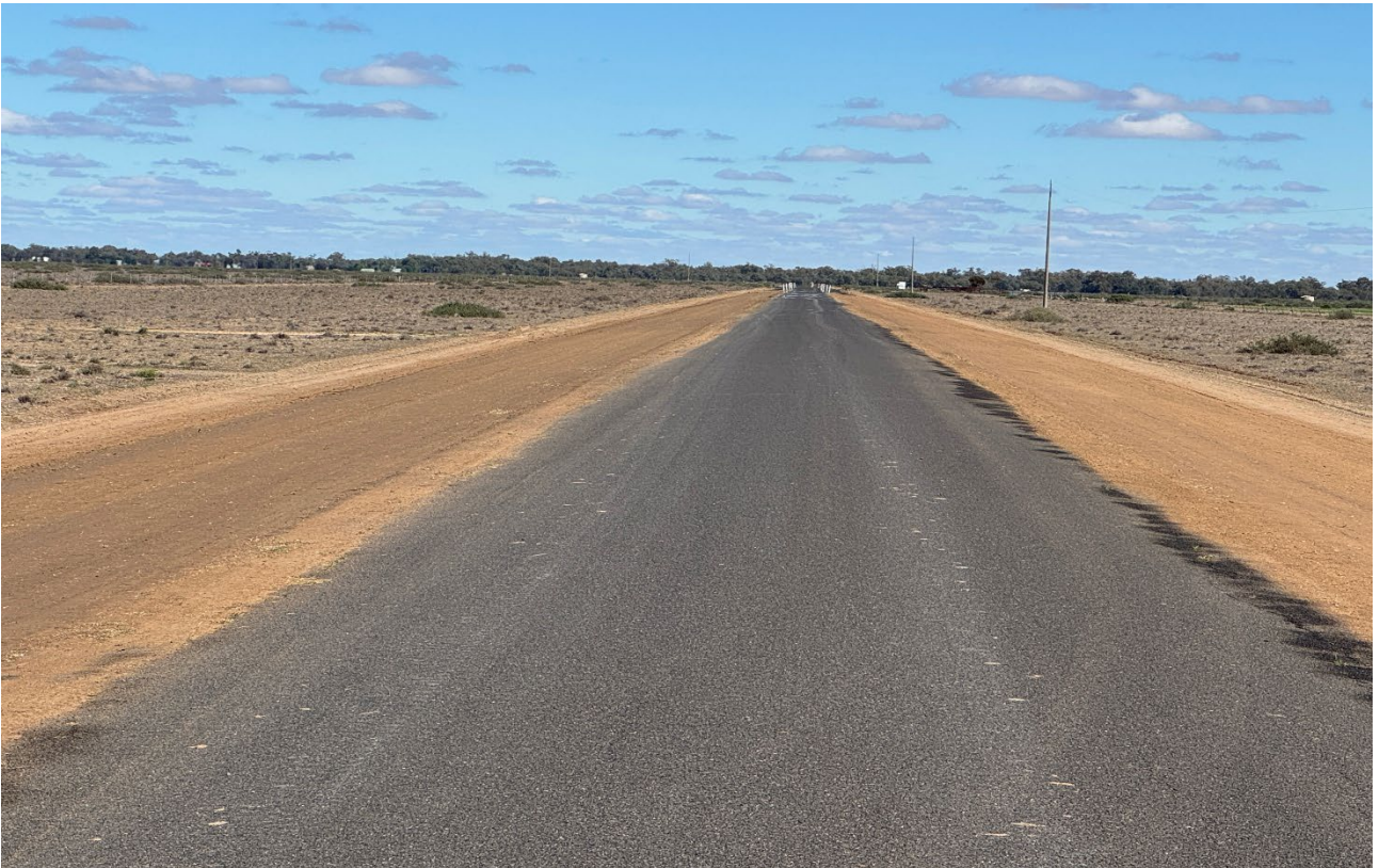
MR501 Shoulder grading
