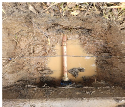
Filtered water repair piper street
