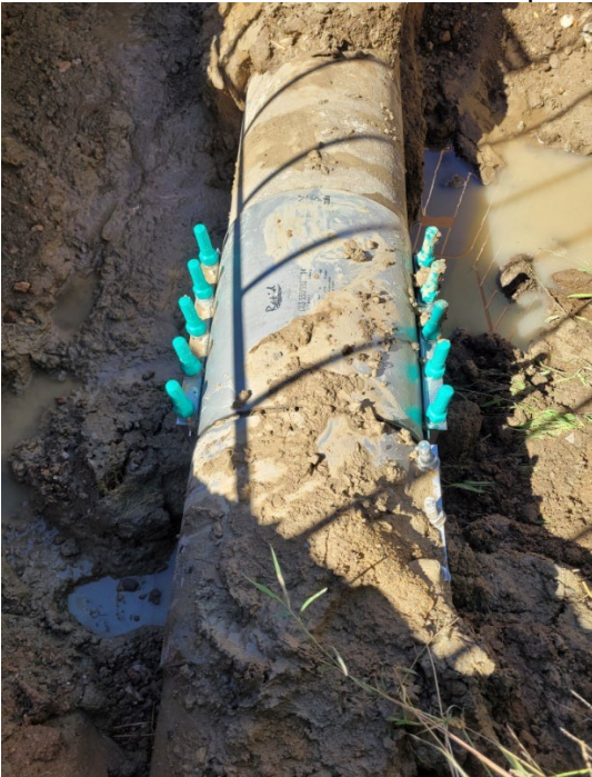
300mm raw water main repair
