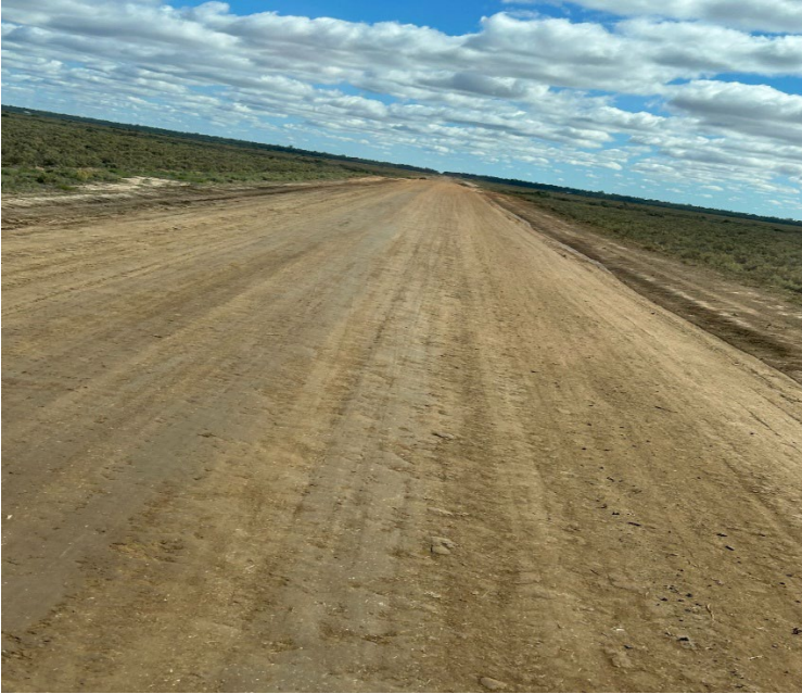
Maintenance grading – Booligal/Gunbar Road
