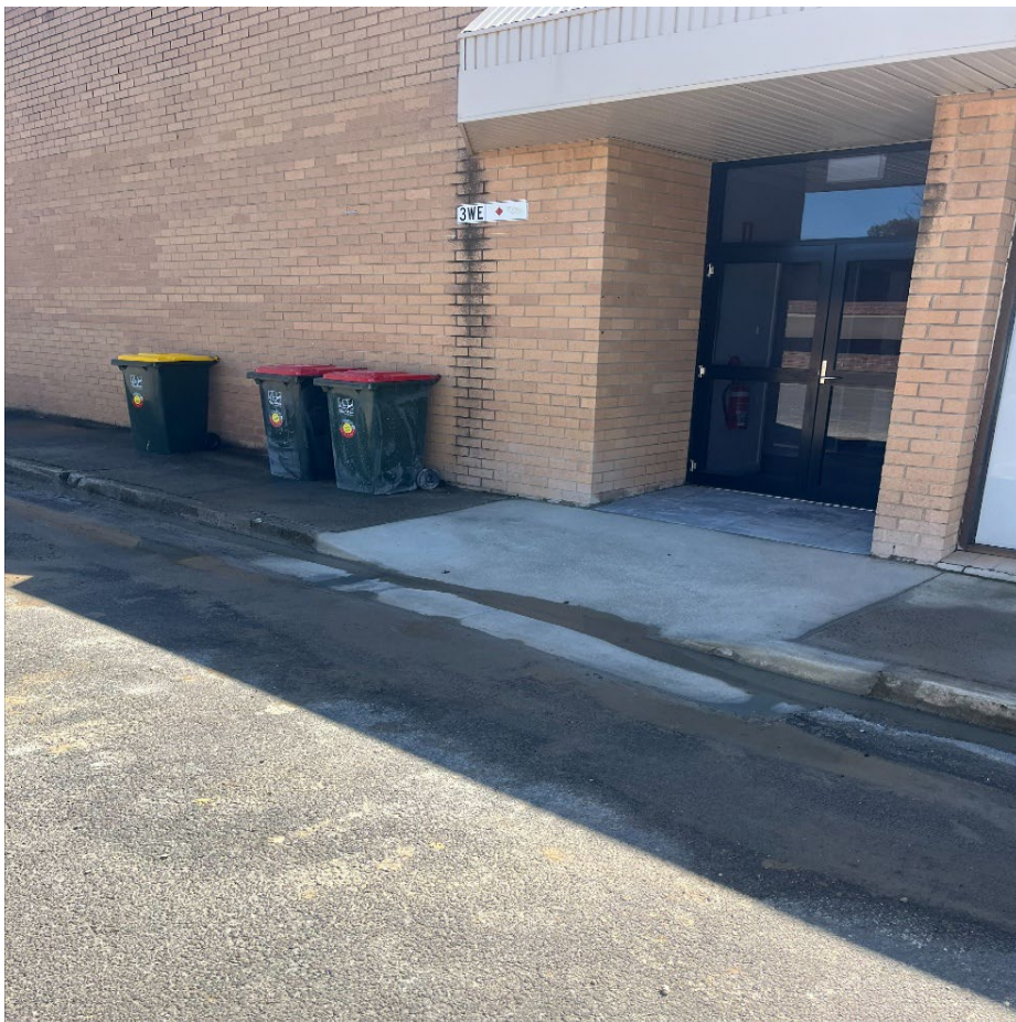
New accessible ramp in Moss Street
