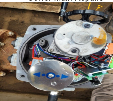
Repairs to actuator at Leonard St Reservoir
