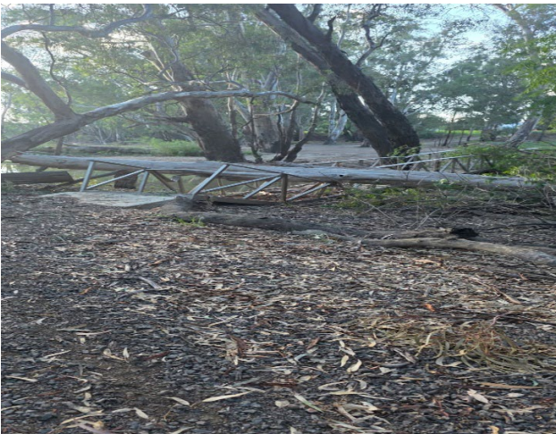
Madman's Bend footbridge damage from fallen gum tree
