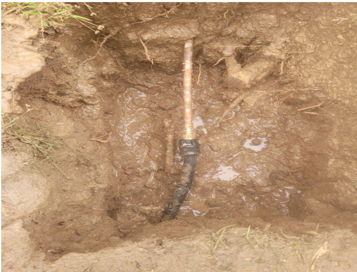
Service connection repairs
