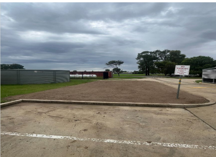
Hardstand area to Hay High School
