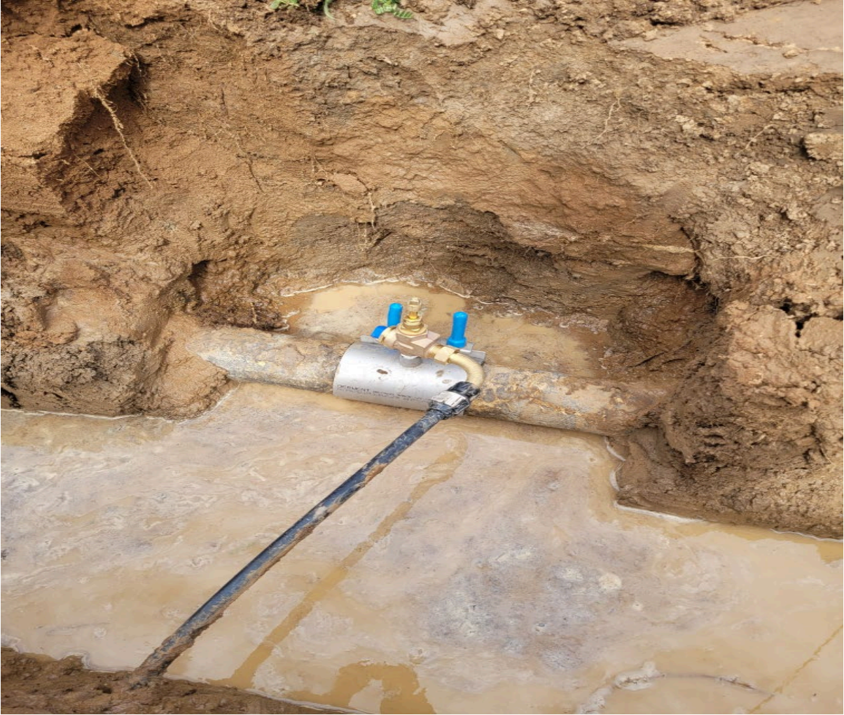
100mm Raw water main repair
