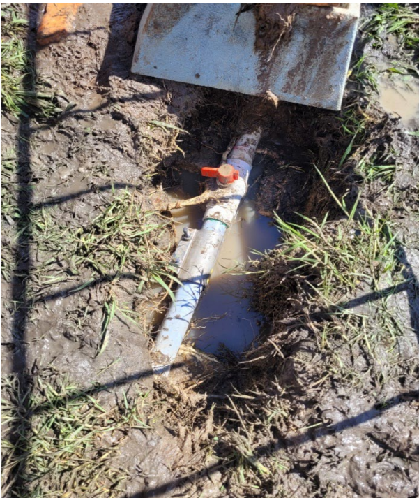
50mm filtered water repair
