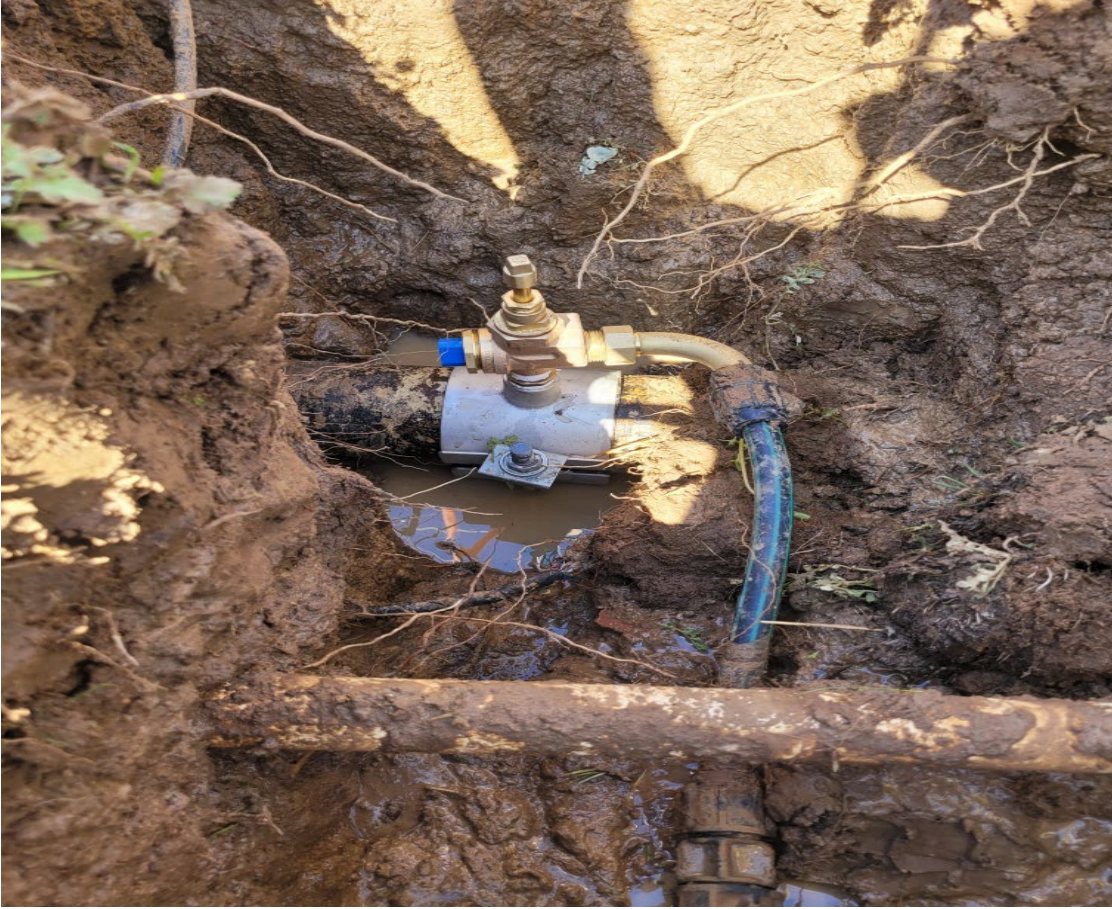
100mm Raw water main repair
