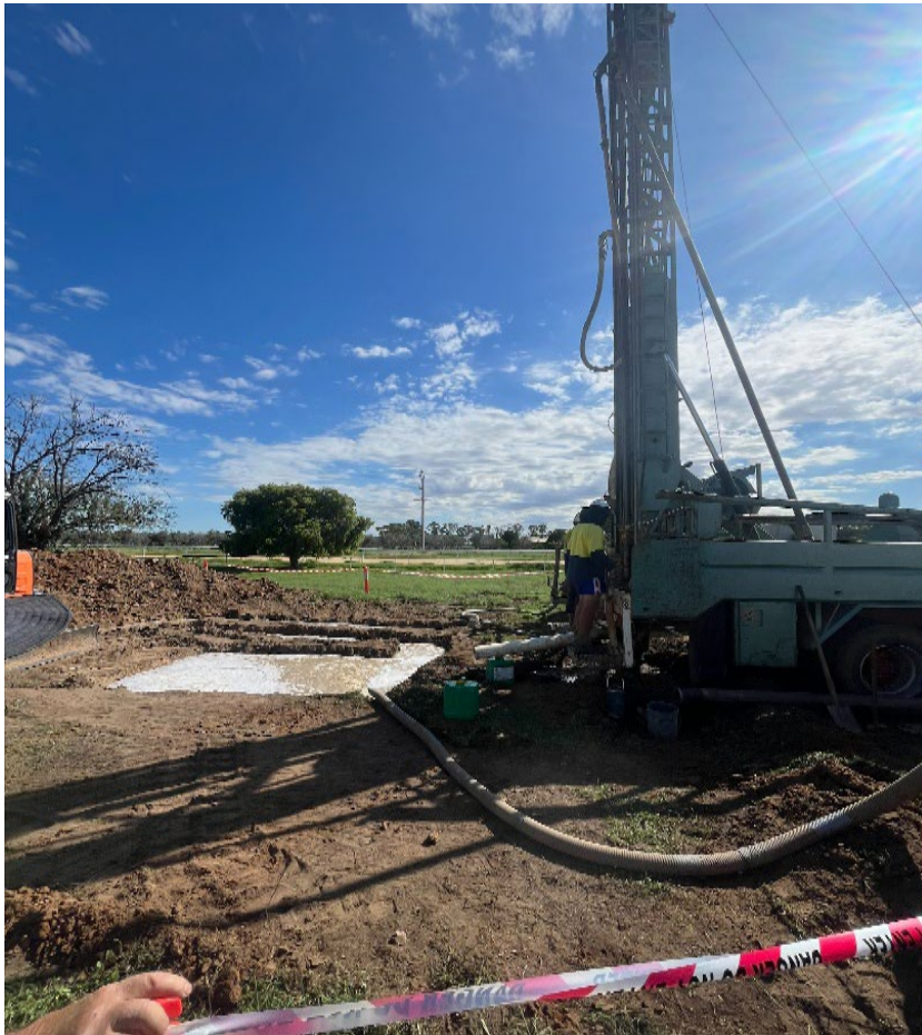
Showgrounds bore water drilling investigations
