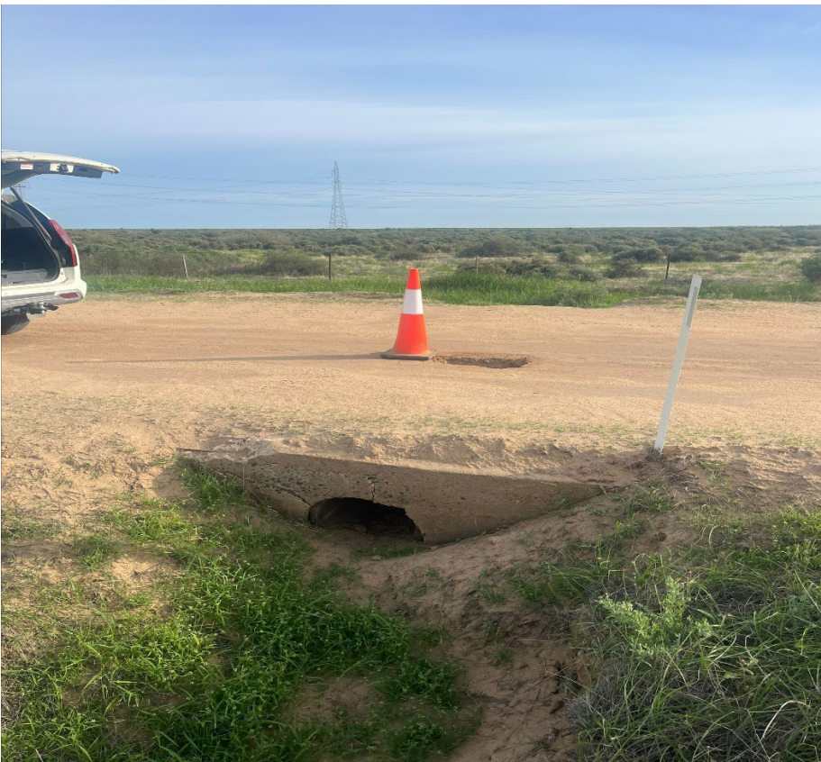
Culvert repairs – West Burrabogie Road
