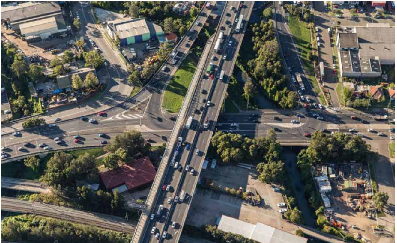
Aerial photo of M4 Motorway and James Ruse Drive at Clyde, Sydney
