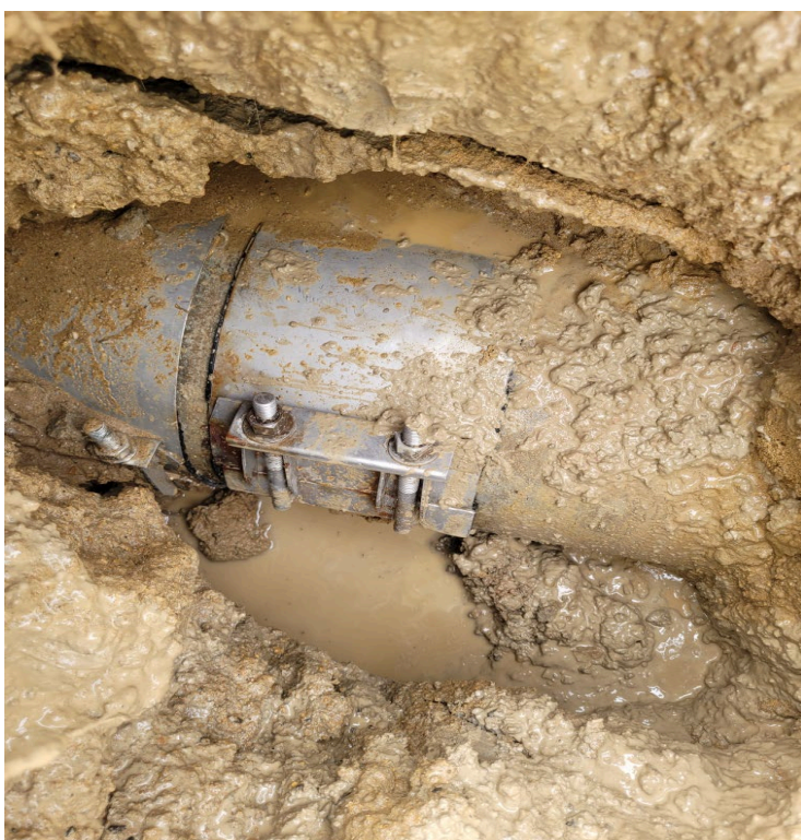
300mm Raw water main repair
