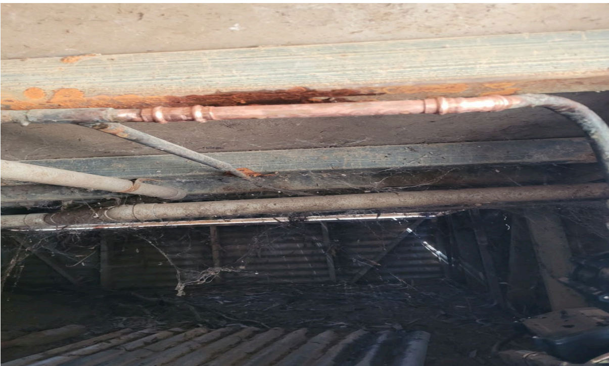
Sandy point pipe and pump repairs
