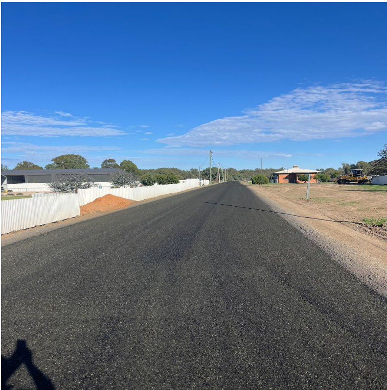
Brewery Street upgrade
