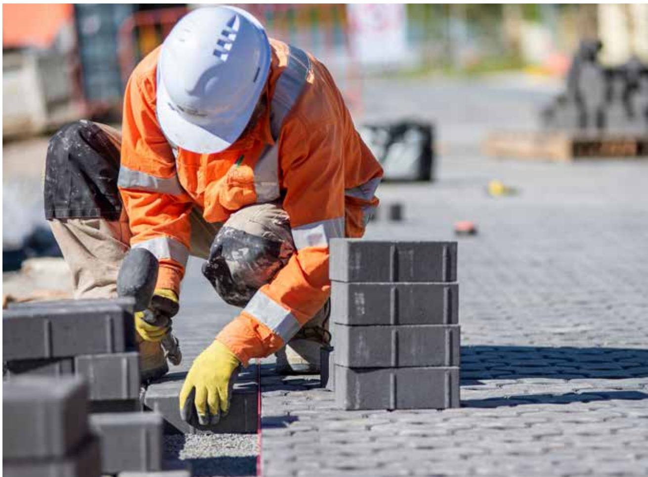
Construction worker laying bricks for footpath
