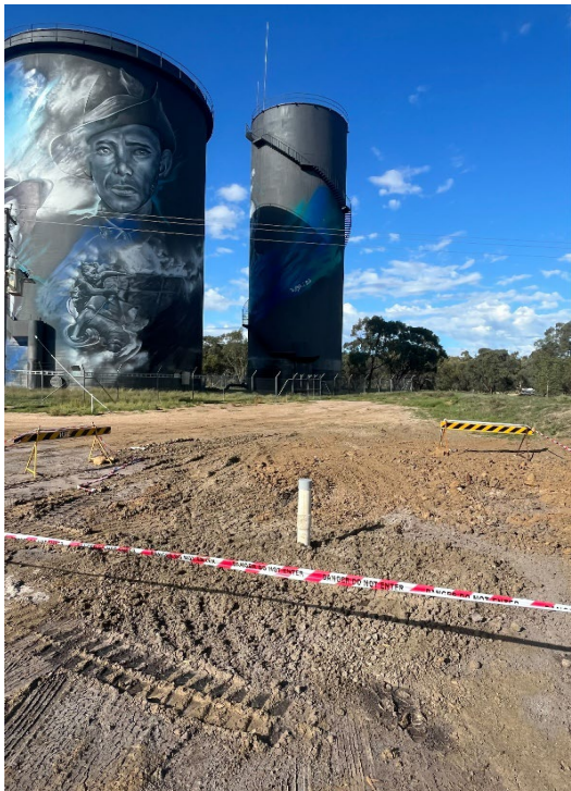
Pine Street bore water investigations
